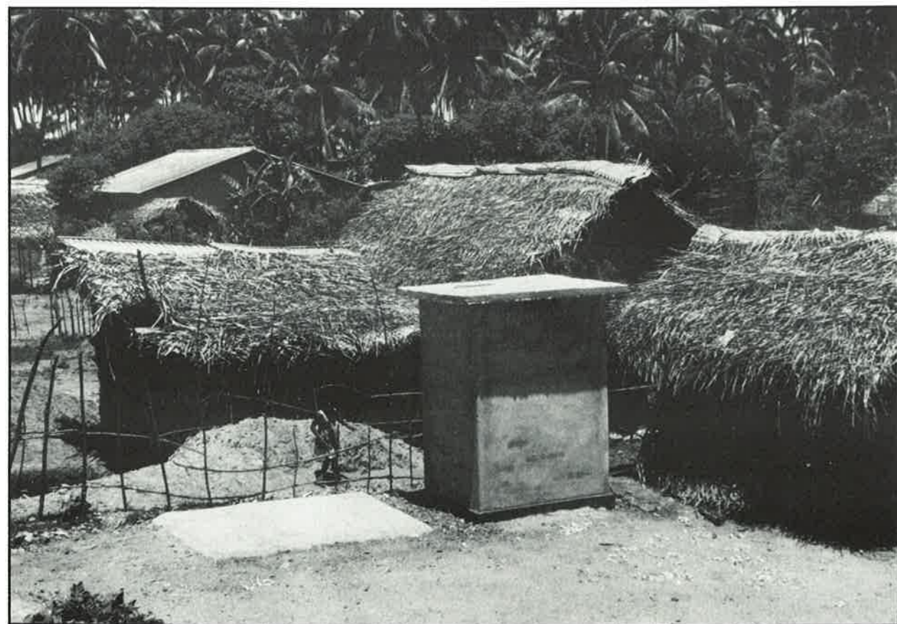
Below: The householder builds his latrine with aid of a loan before commencing house construction
