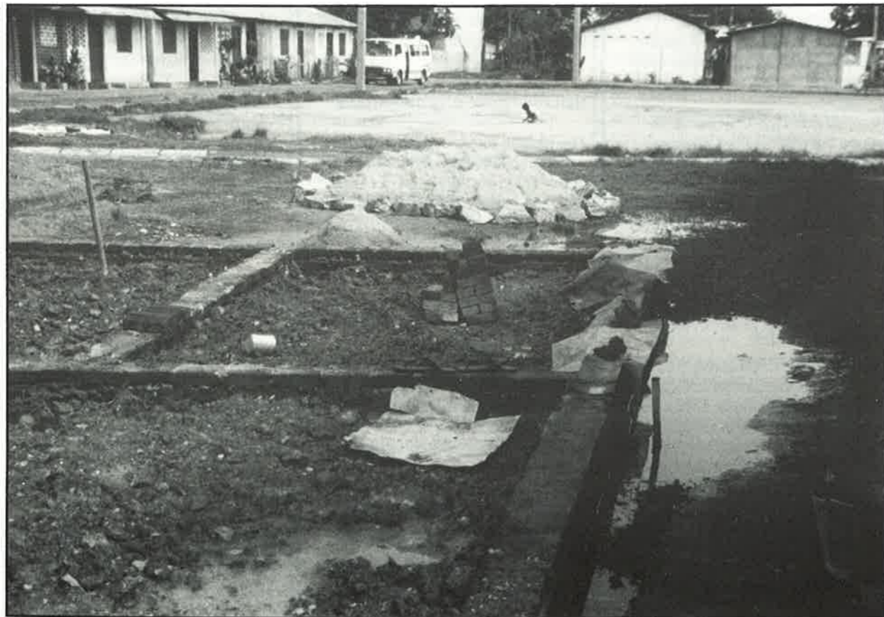
Below: A site prepared without adequate gradient or drainage
