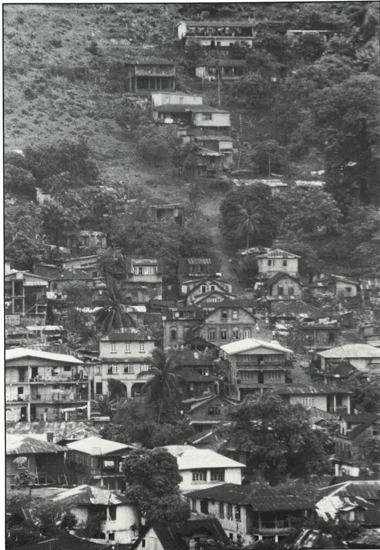
Above: Buildings on a steep slope
