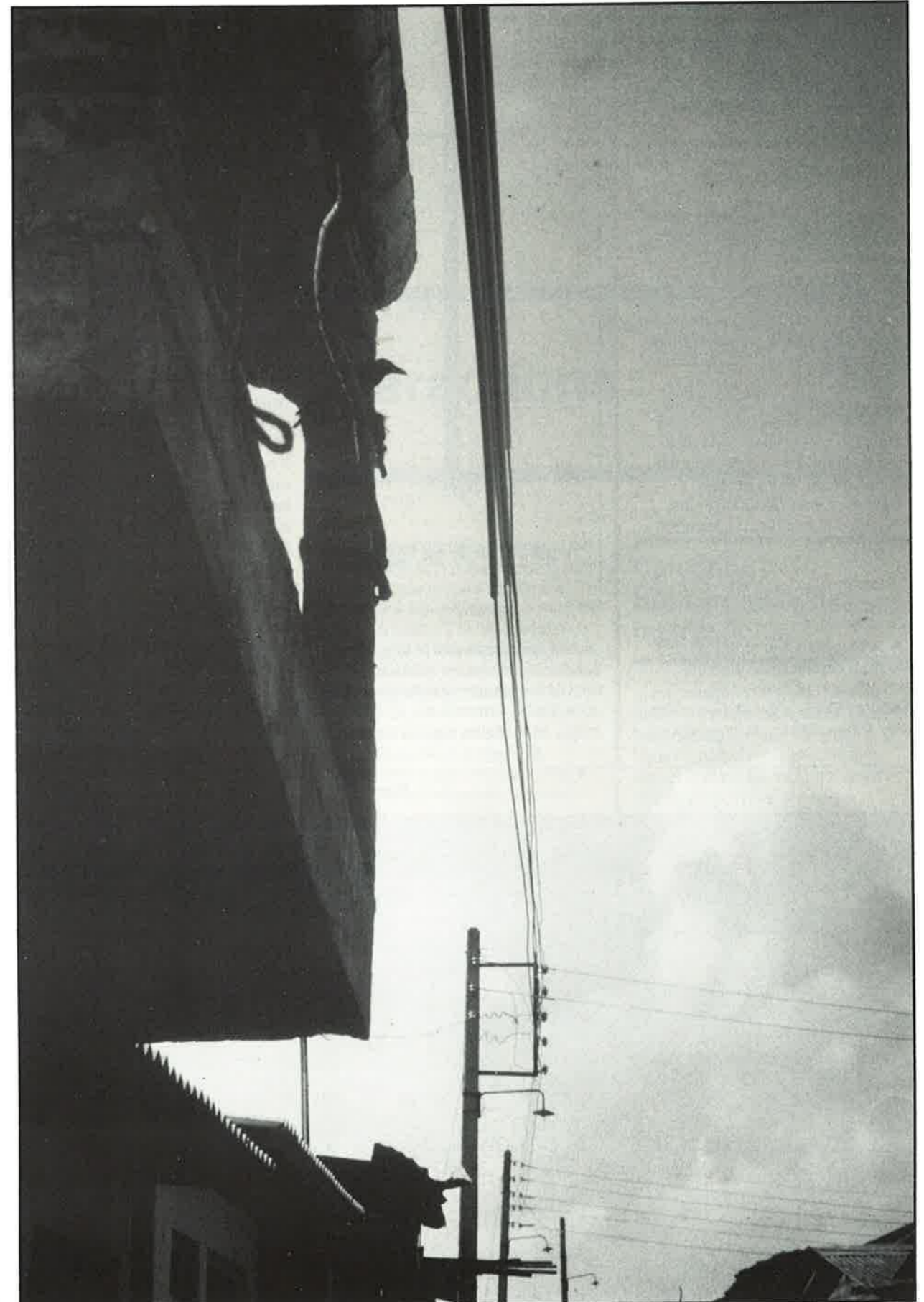
Above: Problems of community housing design clashing with the safety needs of utilities
