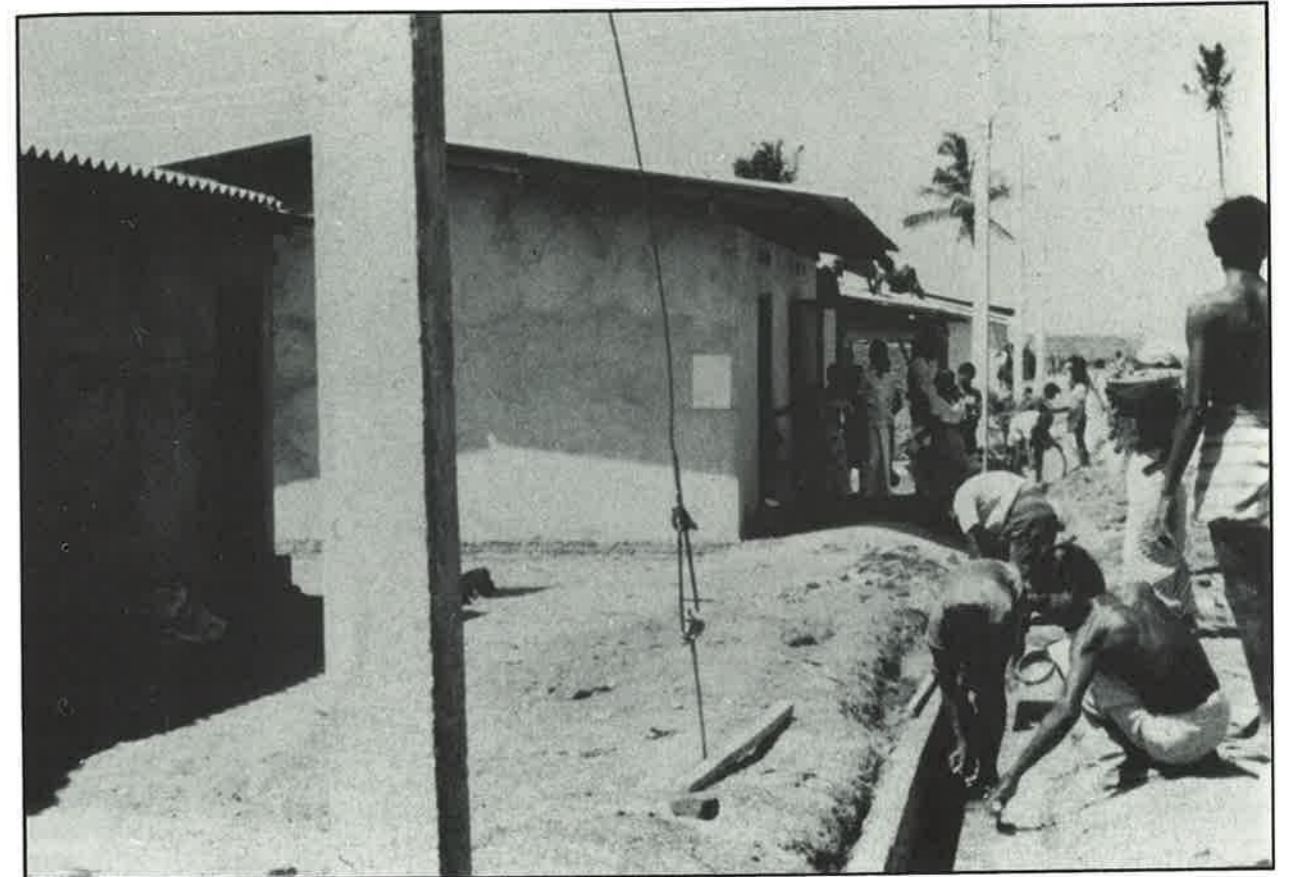
Above: Rectangular section open channel drain under construction
