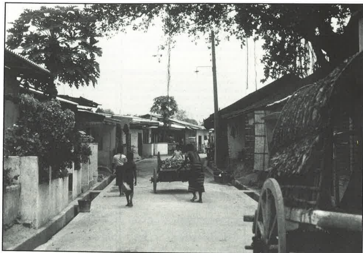
Above: Bitumen surfaced cluster access clearly defined by drains
