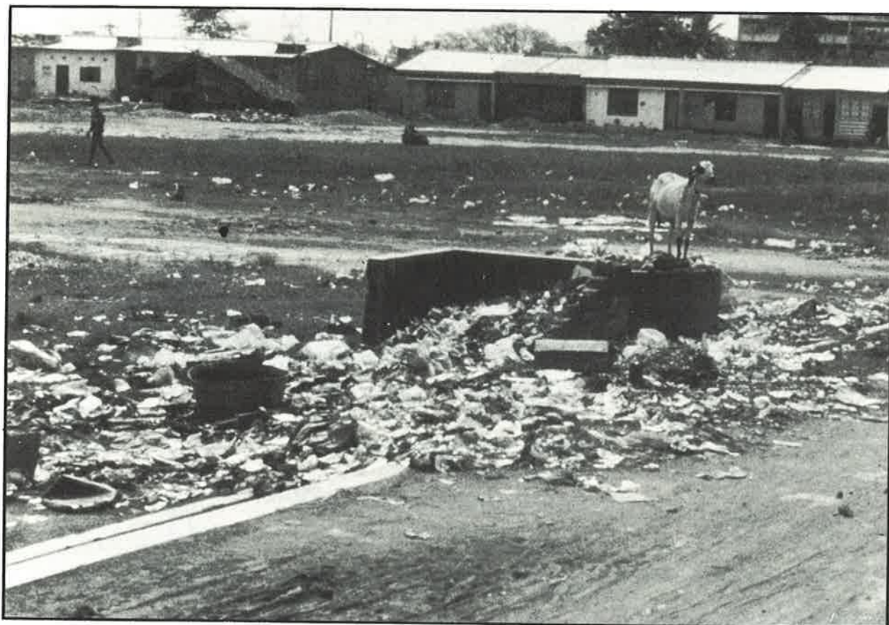
Above: Solid waste spills out and blocks the drains due to incorrect siting of the enclosure and infrequent emptying
