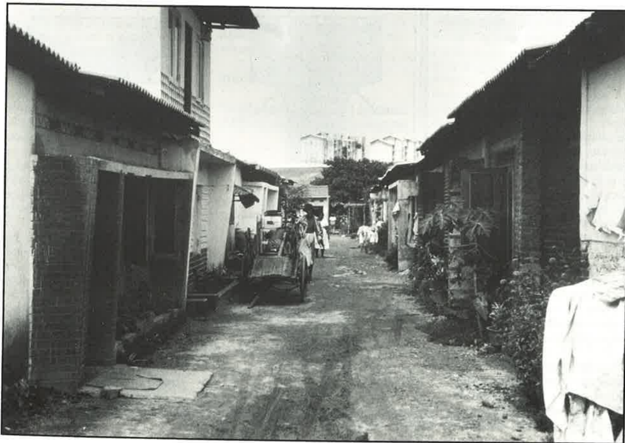
Below: An economical cluster access road
