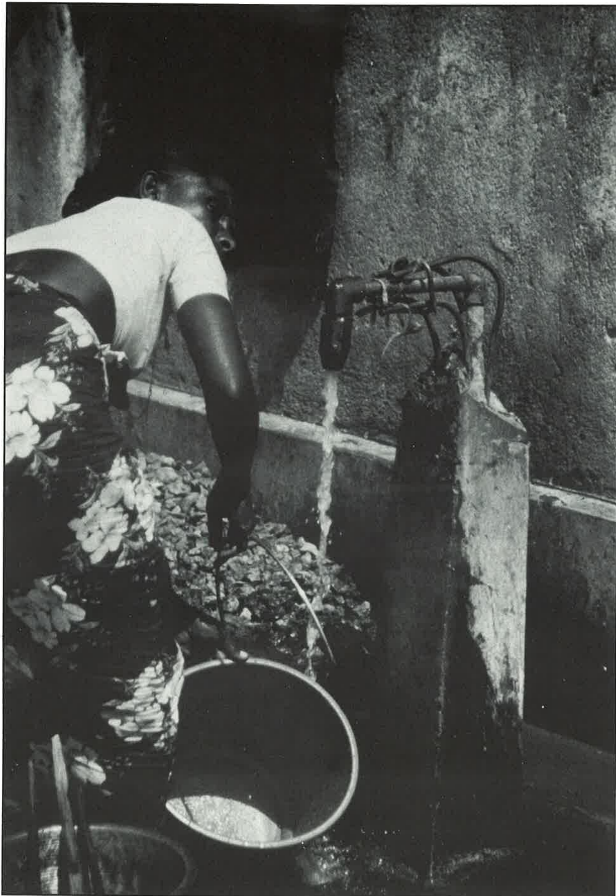
Above: The tap is still working but maintenance is required
