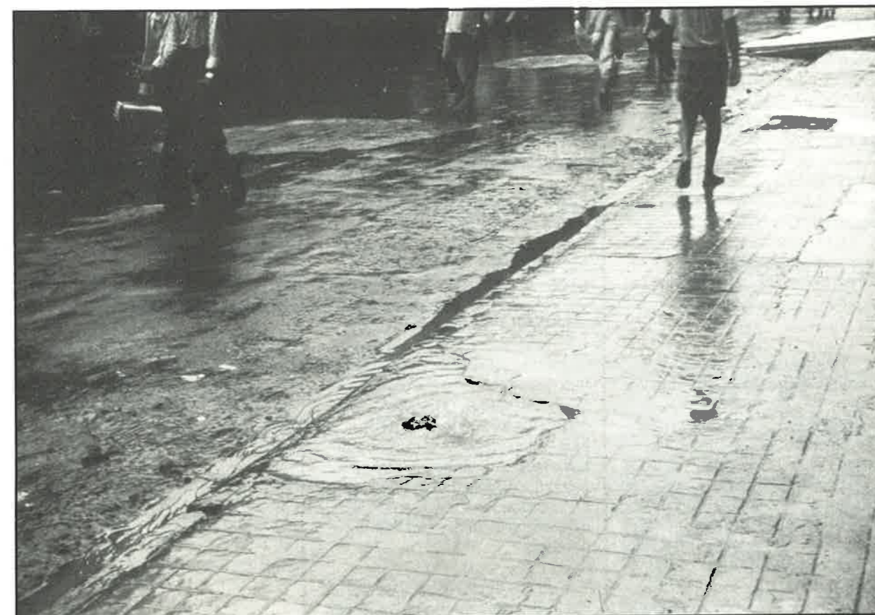
Below: Water is wasted from an unmaintained standpost which has been broken off and removed
